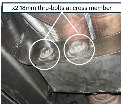
Figure 11d: Cross-member bolts
