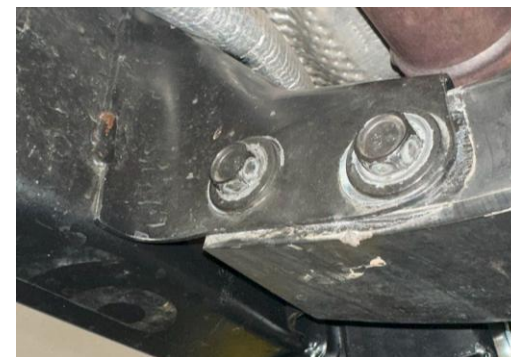
Figure 10: Cross-member bolts flipped around
