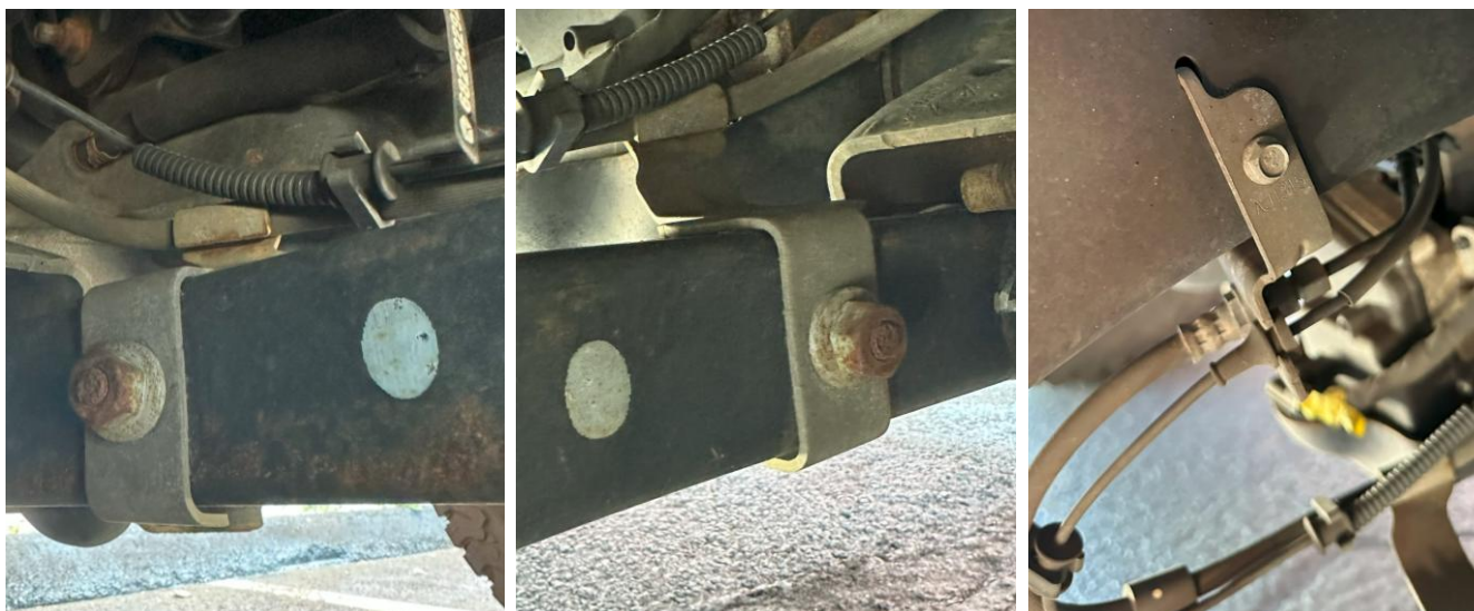
Figure 15: Brake line brackets reinstalled
